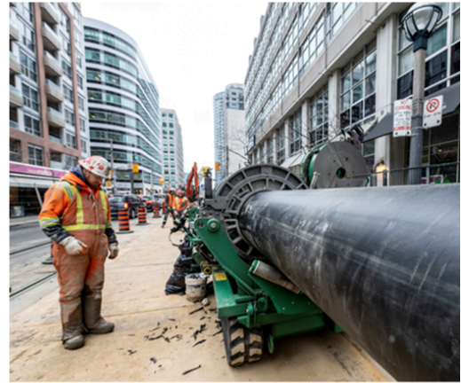
Enwave distribution piping being installed on Blue Jays Way
